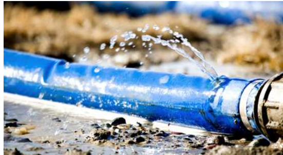
Illustrative example of water leakage
